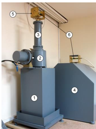
Figure 1. Standard facility for realization of lightning impulse current unit
